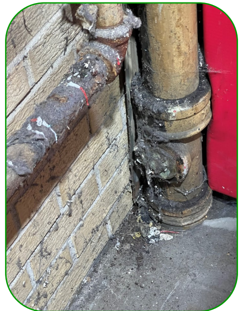
Photos of the old insulation wrap & tape & the dirty, dusty pipes ↓
