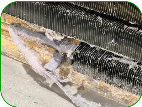
Photos of the very dusty & dirty radiator coils behind the red vent covers →
